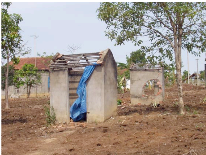
Picture 10: Latrines in a resettled village
