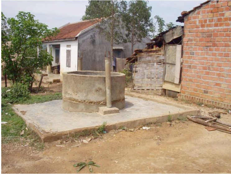
Picture 11: A dry well
