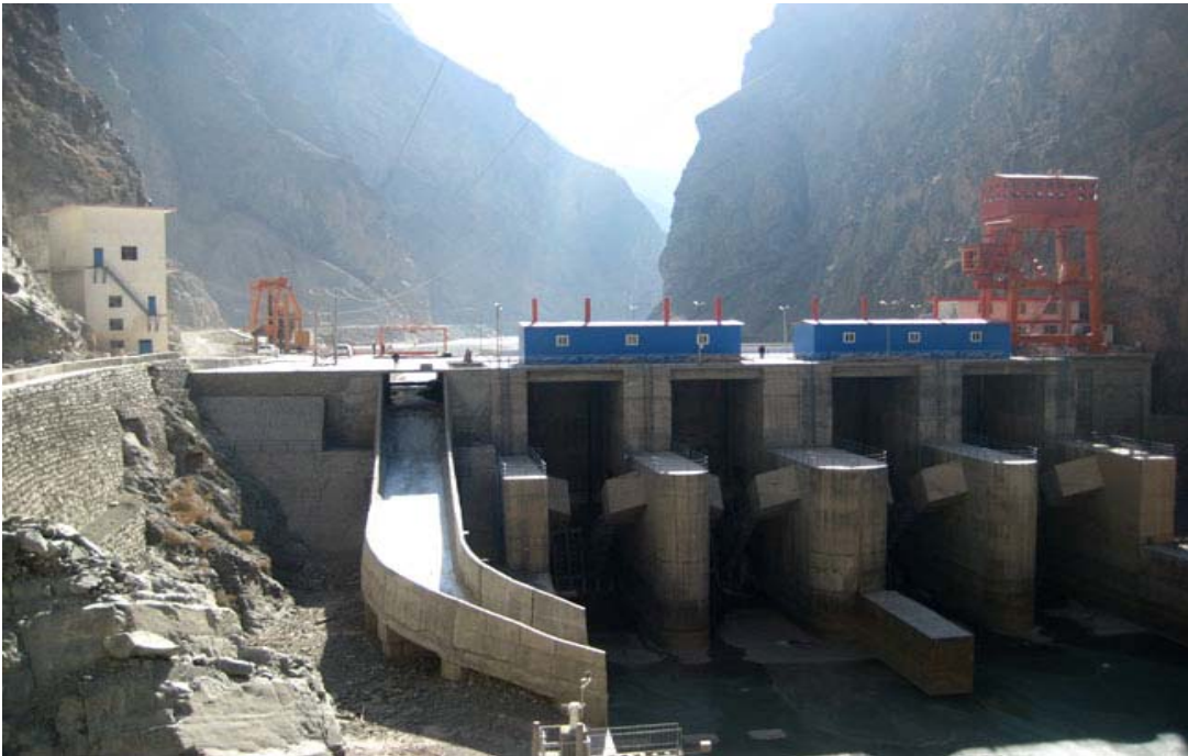
Xiaogushan Hydropower station, Gansu province
