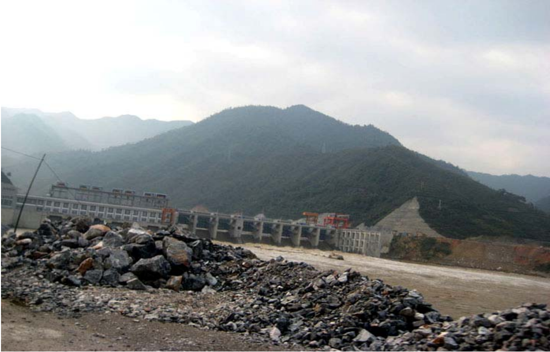
Xiaoxi Hydropower station, Hunan province
