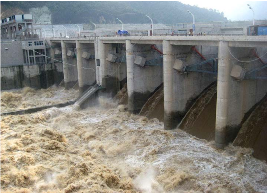
Xiaoxi Hydropower station, Hunan province
