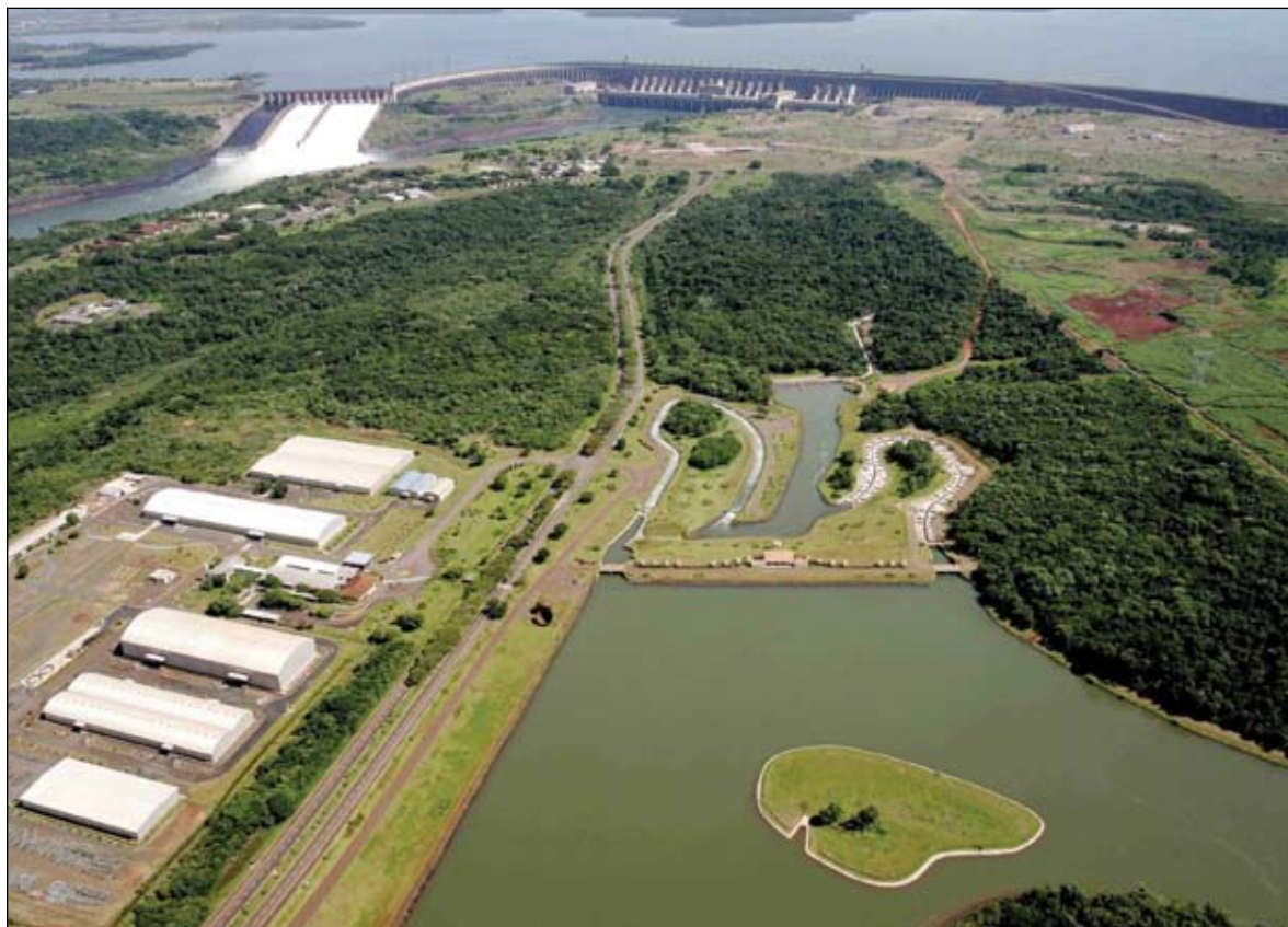
The elaborate fish passage at Itaipu Dam is being used as a model for new dams in the Amazon, but its effectiveness has not been proved. Photo: Caio Coronel/Itaipu Binacional
