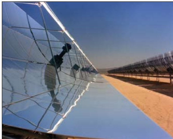
A line-concentrator solar power plant in the Mojave Desert, California. Oil in the receiver tubes collects the concentrated solar energy as heat. The hot oil is then pumped to a power block located at the power plant for generating electricity. Photo: Warren Gretz
