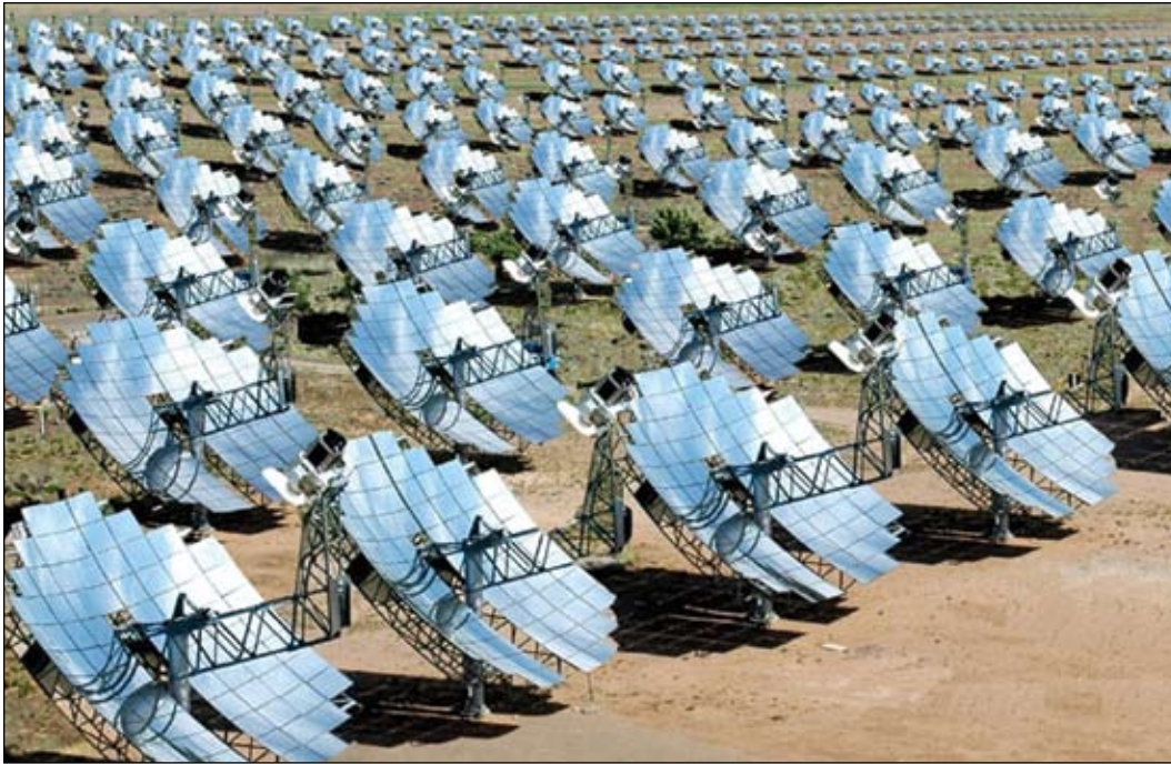
Dish Stirling solar power systems concentrate the sun's heat to run a Stirling engine, which drives an electric generator. This highly efficient solar energy production system also can use alternative fuels instead of the sun's heat so power can be made day or night.
