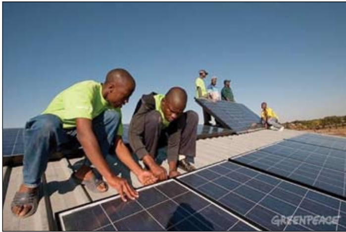
South African high school students install solar panels on their school's roof. Photo: Nicolas Fojtu/Greenpeace
