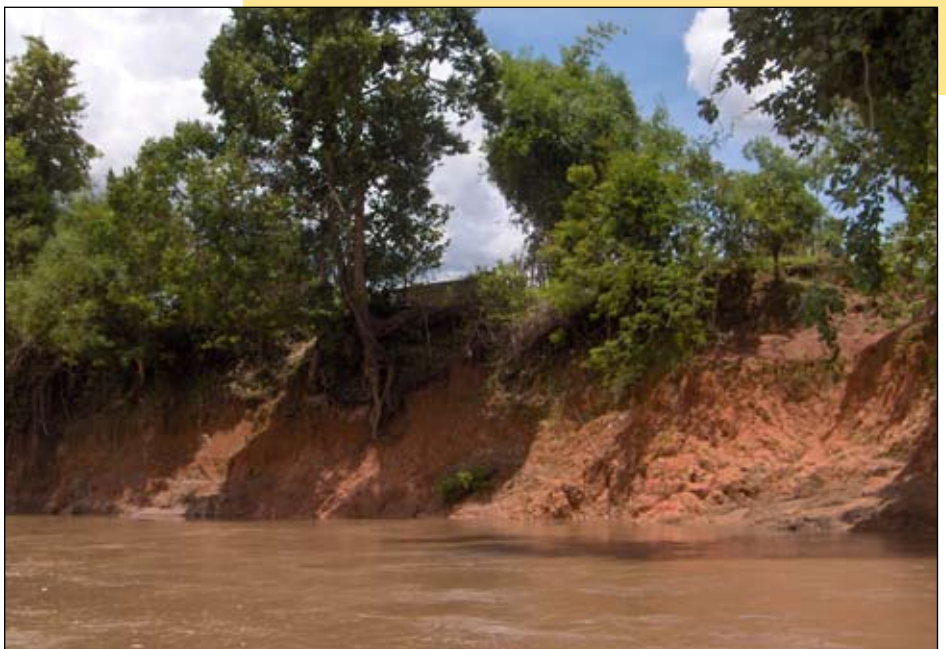
Erosion along the Hinboun River. Photo: Vinya Sysamouth
