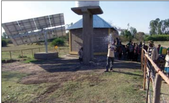
DWC helped implement this solar pumping station in Ethiopia.
