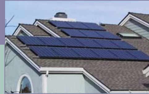
Rooftop solar grew leaps and bounds in 2011. Photo: Akeena Solar
