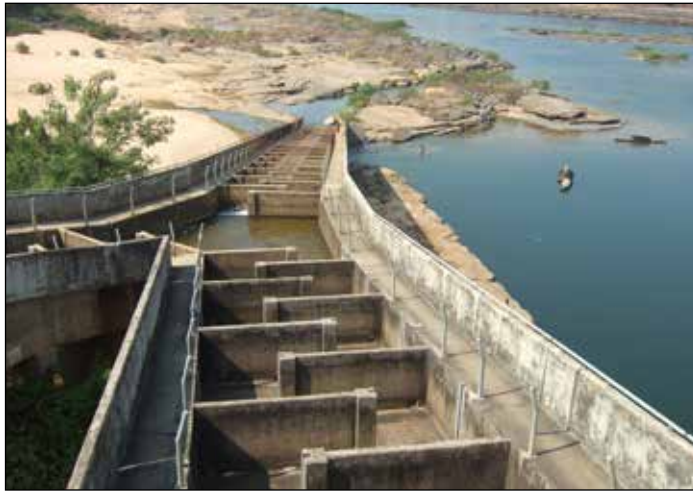
The failed fish ladder at Pak Mun Dam. Photo: David Blake
