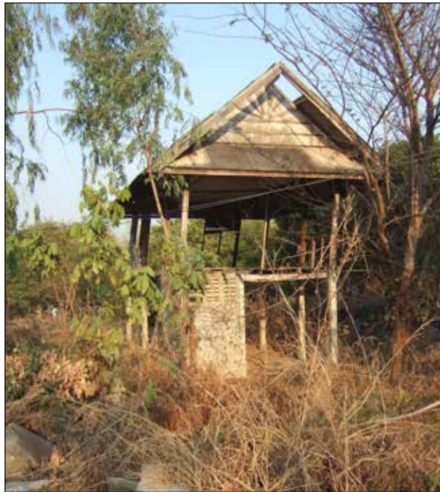
An abandoned resettlement house at a village that was forced to move for Pak Mun dam and now stands testament to its failed resettlement process. Photo: David Blake
