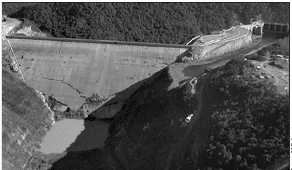
Campos Novos Dam in Brazil (shown here after cracking led to uncontrolled emptying of its reservoir last year). This 880 MW completed project is seeking CDM credits.
