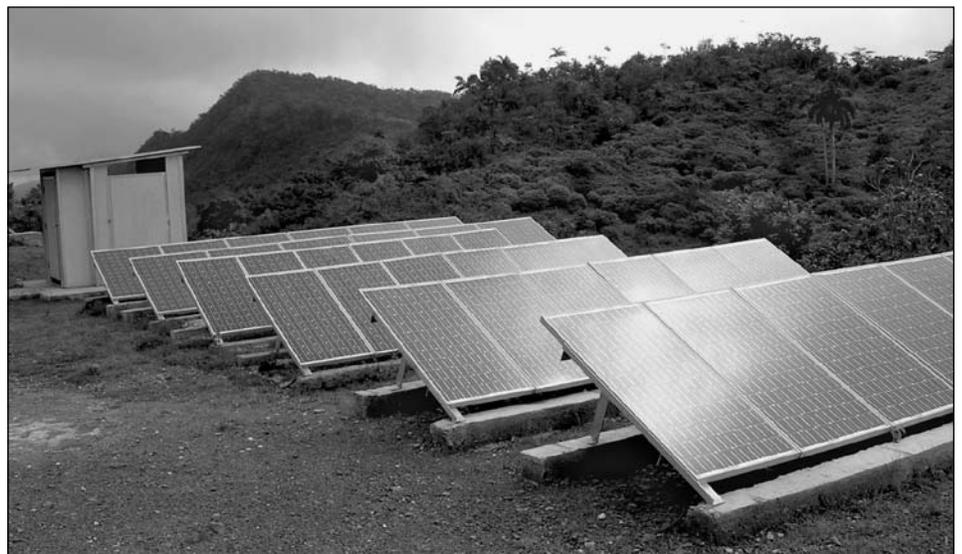
Solar panels in Cuba's "Cuchillas del Toa" biosphere reserve. These panels provide electricity for the forest keepers' buildings.
