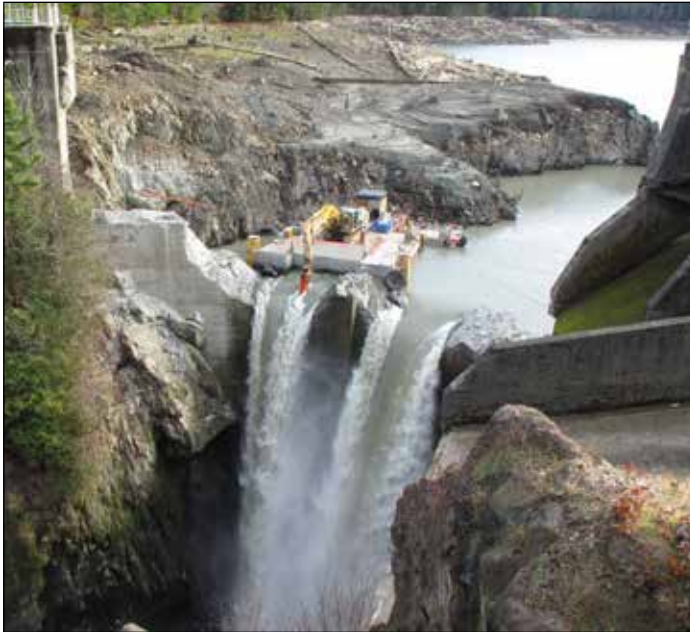
Removal of Glines Canyon Dam on the Elwha River has resumed after a year's hiatus. Photo: Lower Klallam Tribal Library
