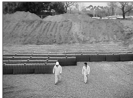
Field infiltrators being installed at Broadous School.
