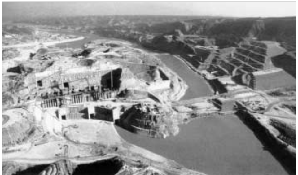
Xiaolangdi Dam under construction.
