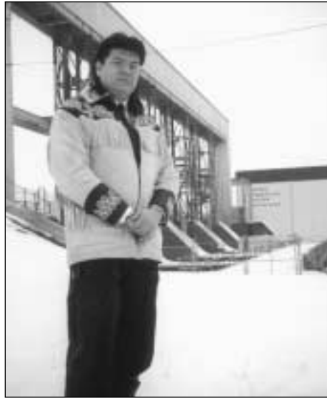
Chief John Miswagon, in front of the Jenpeg generating station near Cross Lake.
