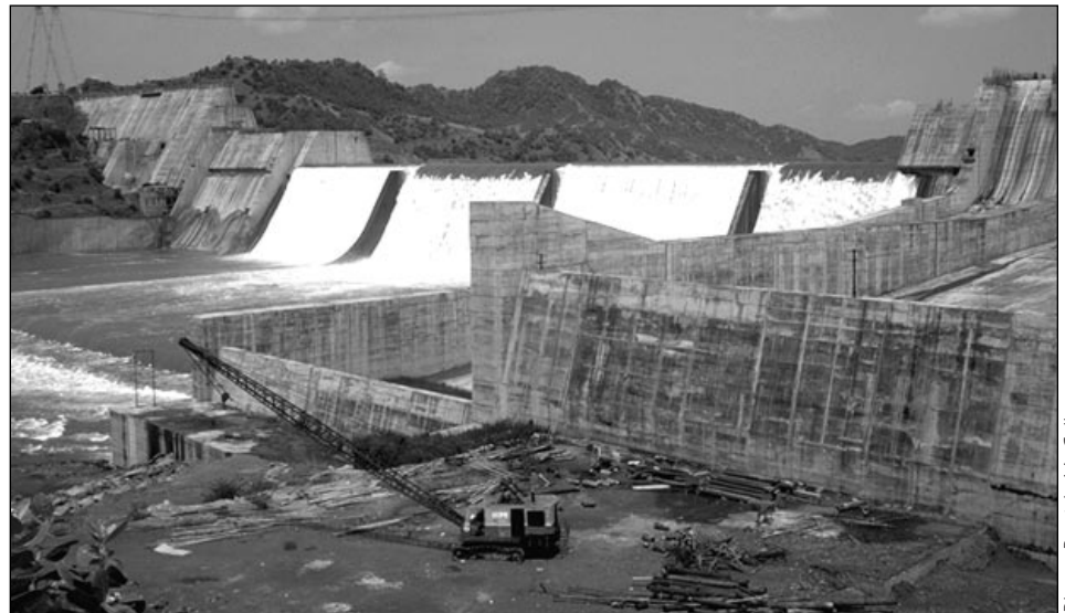
The Sardar Sarovar Dam under construction.
