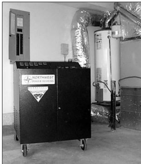
This prototype fuel cell unit can power a typical 3-bedroom house in the US. Photo: NPS
