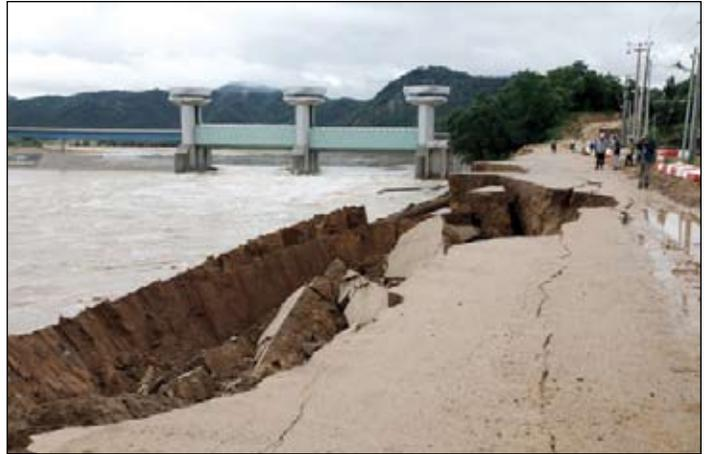
The newly completed levee near Sangju Dam, part of the Four Rivers project, collapsed on June 25, 2011. Water flows throughout the river have changed due to flaws in dam design. Environmental experts expect problems like these to continue. Photo: © Kim/GREEN KOREA
