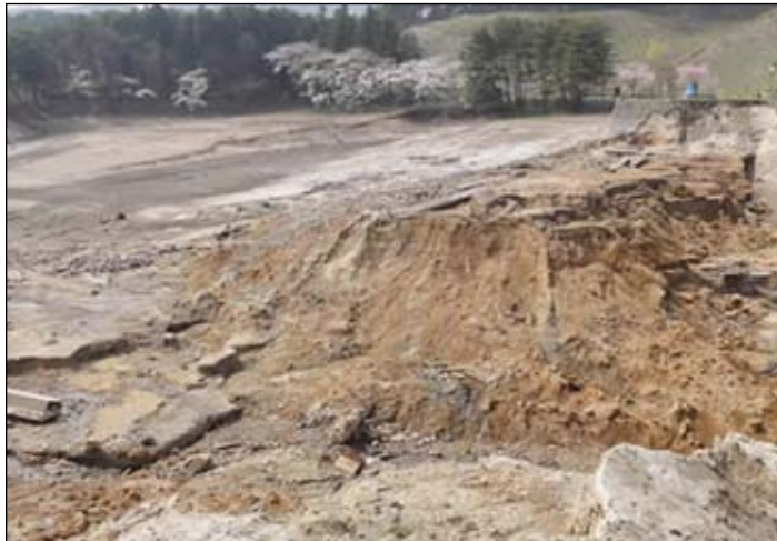
Site of Japan's Fujinuma Dam failure. Photo: Geo-Institute Team
