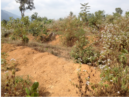
“Terracing” done by THPC for Ban Nongxong canals for Ban Nongxong
