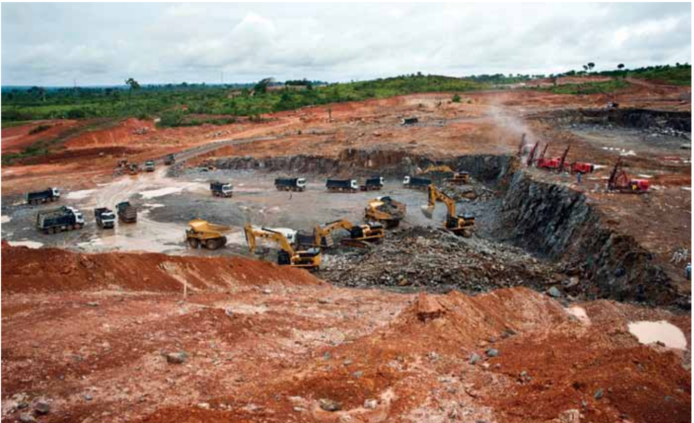
Construction of the Belo Monte Dam, Altamira, Brazil. Foto: Minplanpac
