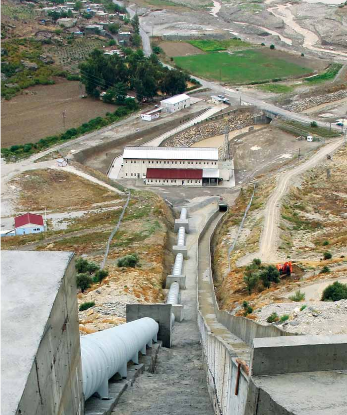
Statkraft's Cakit Hydropower Plant, Turkey. Photo: Statkraft
