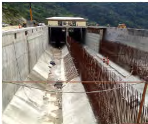
Figure 2-6: De-silting facility under construction at Dagachhu.
