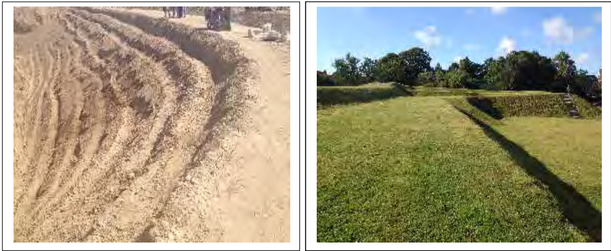
Figure 6-9: Example of muck benching and re-vegetation.
