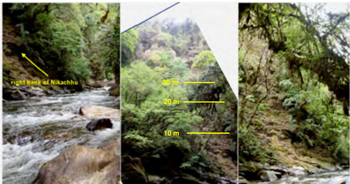
Figure 2-3: Slope conditions at the proposed Nikachhu dam site.
