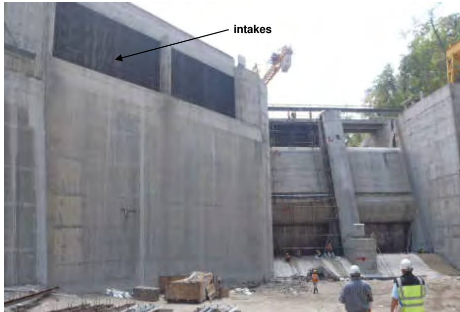
Figure 2-2: Typical concrete gravity diversion dam (at Dagachhu).
