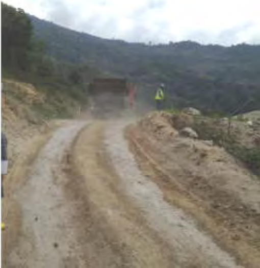
Figure 2-13: Typical access road for a hydropower project (Dagachhu project).
