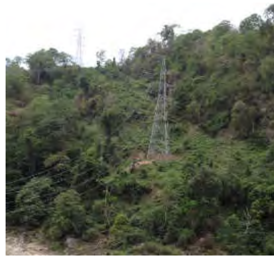
Figure 2-14: Transmission lines at Dagachhu.
