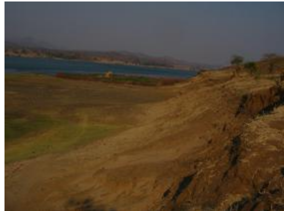
Figure 6.1 Showing erosion of the stream channel downstream of Cahorra Bassa
