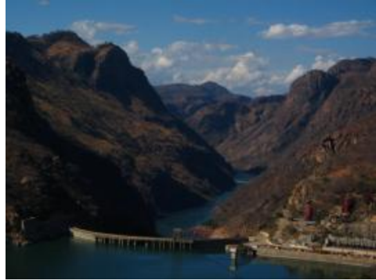
Figure 3.3 Showing the Cahora Bassa Dam Wall
