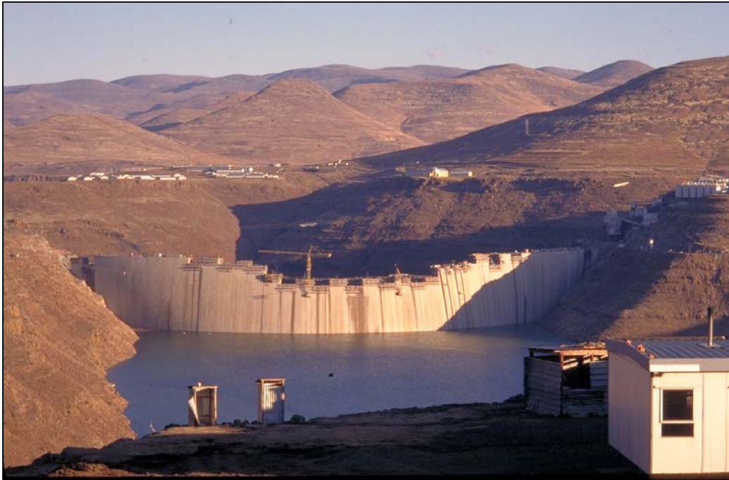
Katse Dam (Lesotho) under construction.
