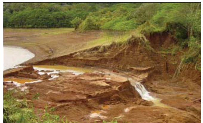
The failure of the Kaloko Dam in Hawaii killed seven.
