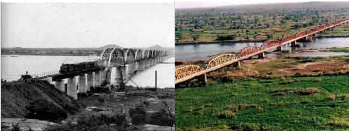
Figure 4: Dona Anna Bridge taken on the same day of the year, but the picture on the left was taken in 1975 and the picture on the right was taken in 1997 26 .
