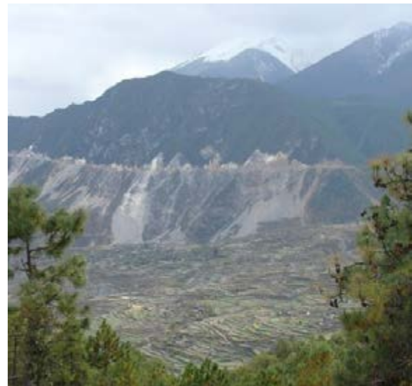
Land slips caused by roads across steep hillslopes
